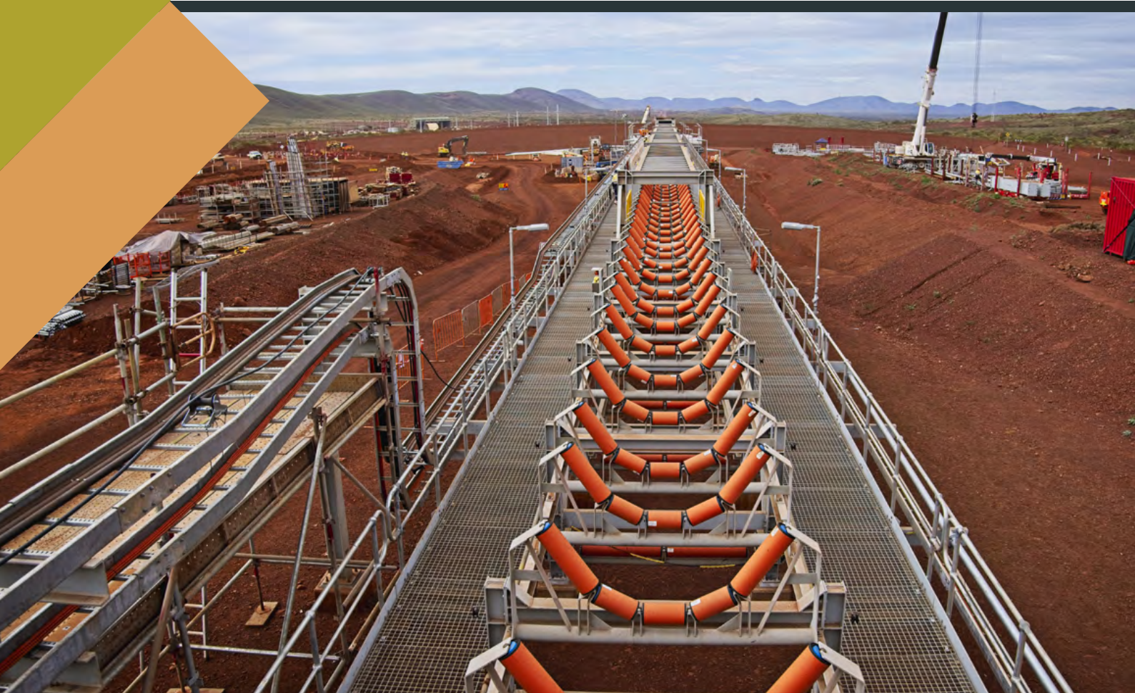
Western Turner Syncline Phase 2 Project, Western Australia
